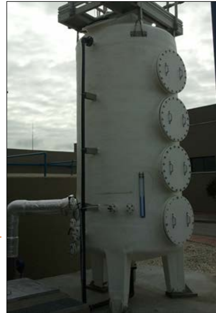
Anoxic desulfurization pilot plant developed by UCA
