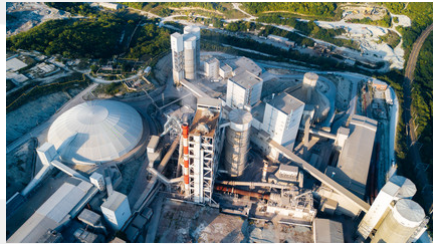
Portland cement manufacture
