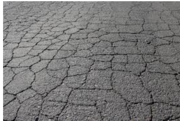
Intermediate T Fatigue Cracking
