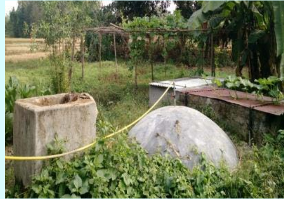
Defunct biogas plant in Napaam
