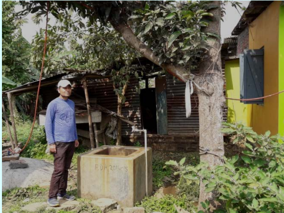
A functioning biogas plant (Amlighat)
