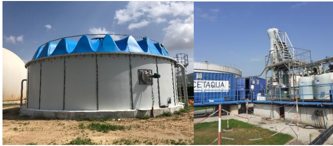
Figure 1 Elutriation tank (700 m 3 ) (left) and pilot P&N recovery units (right) located at Murcia Este WWTP
