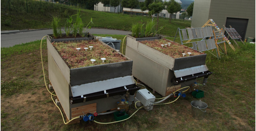
Green roof modules after installation.
