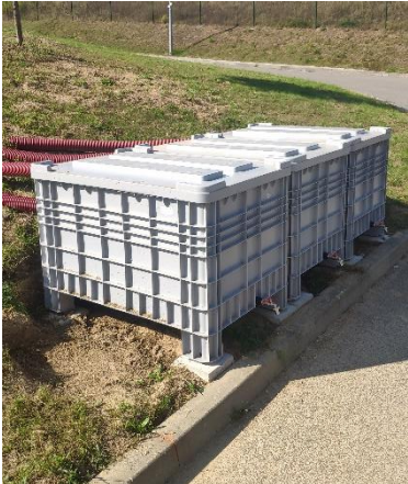
Rainwater storage tanks
