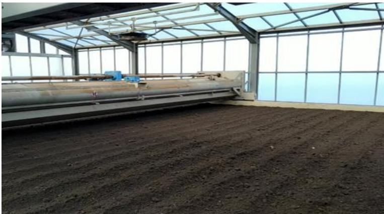
Picture 03: Solar drying unit 02
