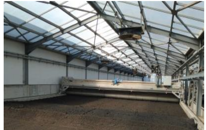
Picture 02: Solar drying unit 01
