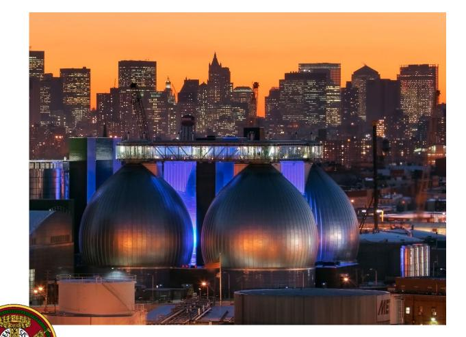
Under standard technologies, only approximately 20-30% of organic matter in the sludge is mineralized, and as much as 70% of the organics remain within. ASD is hence not a complete solution to sludge management, and further treatment of digested sludge is necessary for recovery of remaining recoverable resources.
