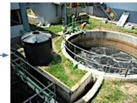
Effluent treatment plant (MBR+RO)
