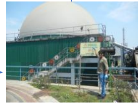
Thermophilic Anaerobic Digester
