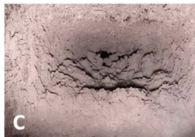
Ash deposits forming during the combustion
