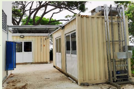
On-site Containerised AD system
