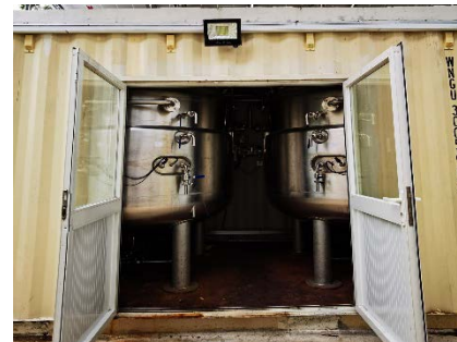
Two main digester
