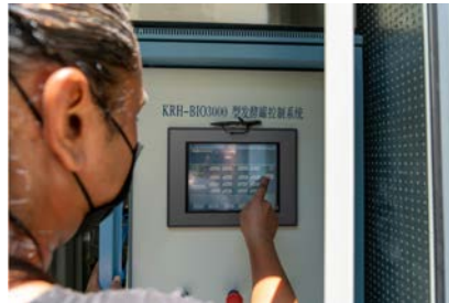
Central control panel
