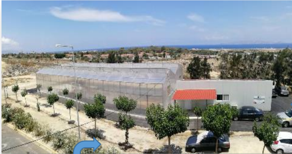
Overview of the Pilot Unit
