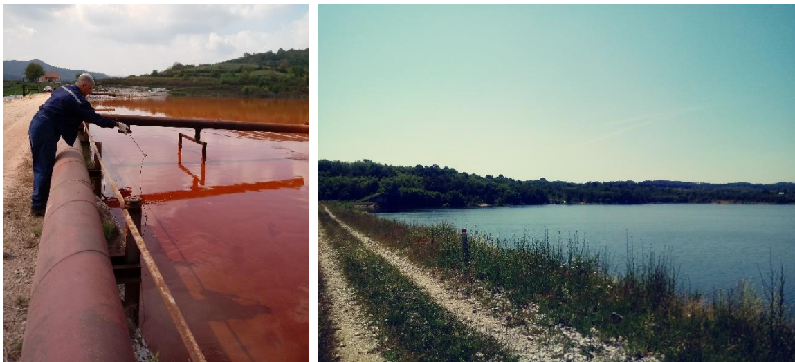
Figure 1. Red mud tailings dam from bauxite processing (left, Zvornik, Bosnia and Herzegovina) and iron mine tailing dam from magnetic separation (right, Prijedor, Bosnia and Herzegovina)
