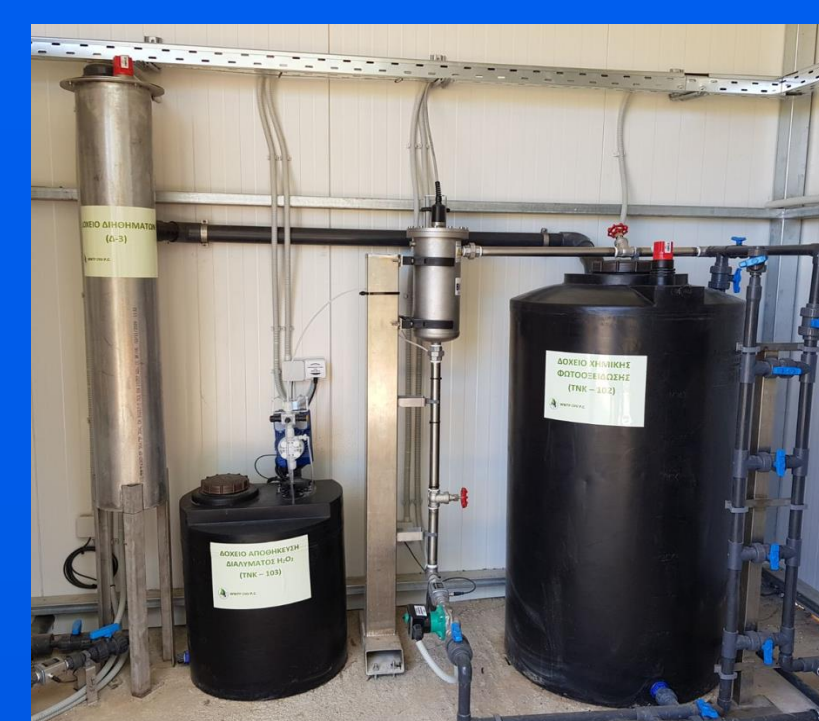
Figure 04: Advanced oxidation unit (UV, H 2 O 2 )
