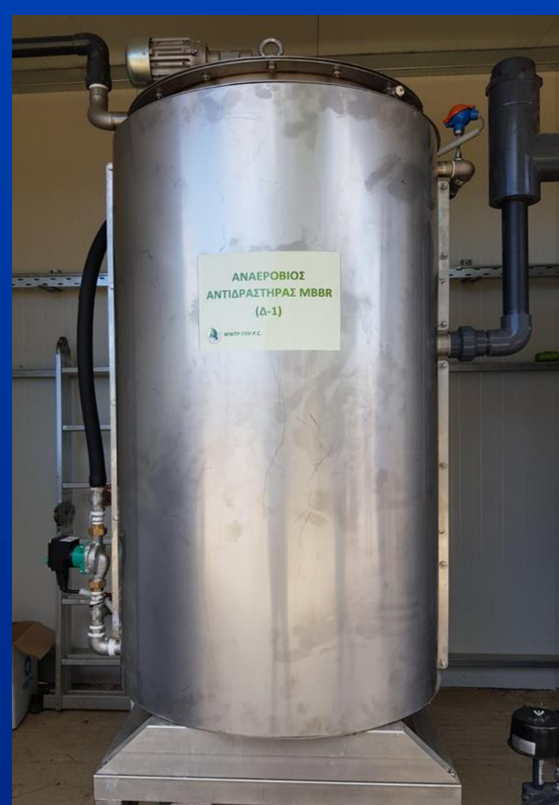
Figure 02: Anaerobic fluidized bed reactor unit (AnMBBR)
