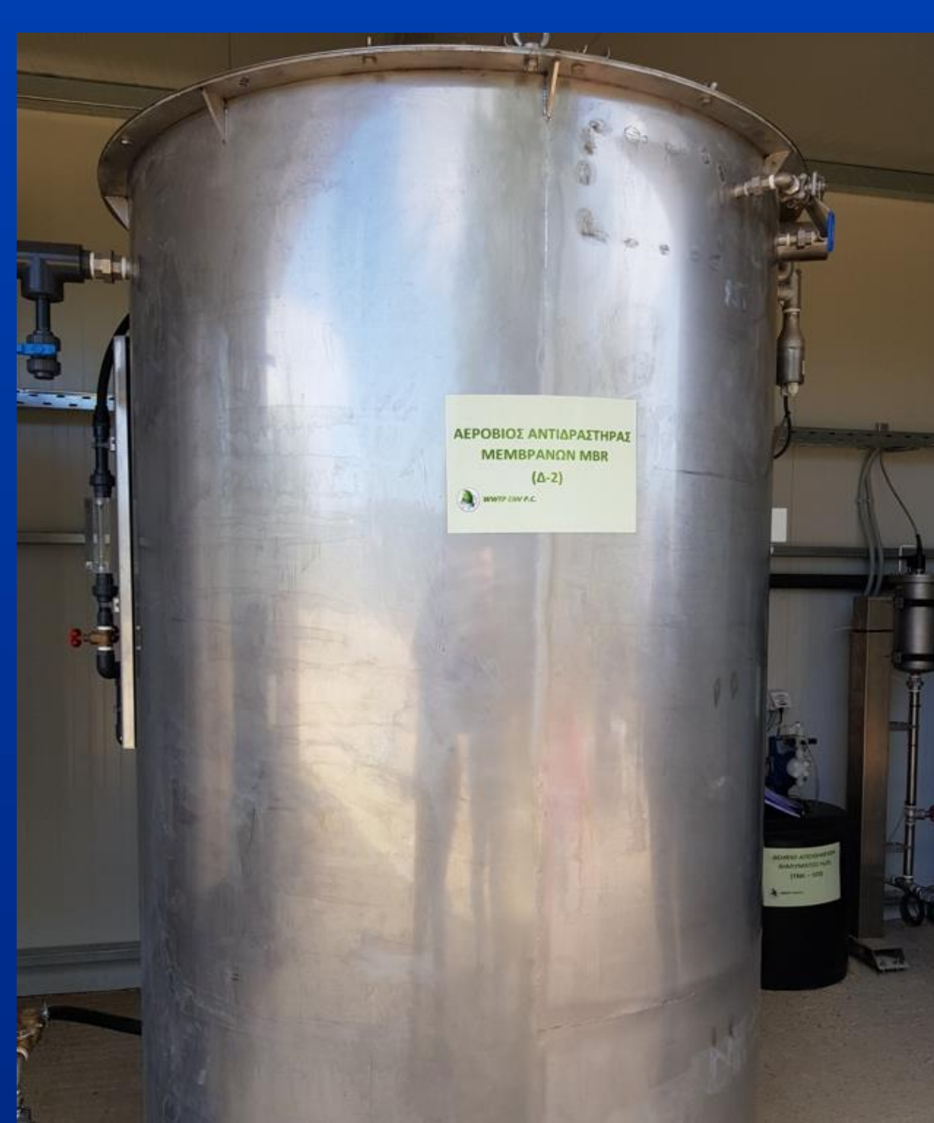
Figure 03: Aerobic biological treatment unit with bio membranes (MBR)
