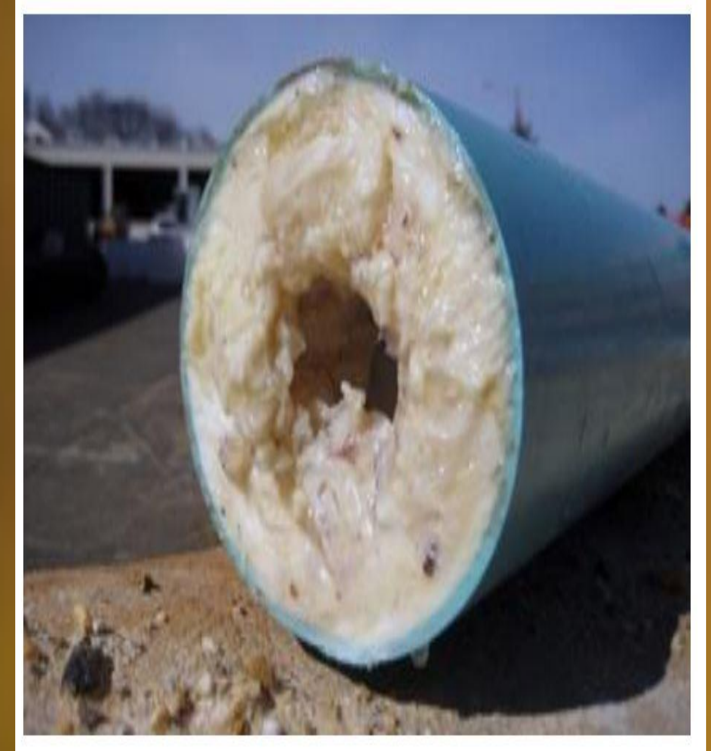
Image of FOG deposit on a sewer pipe wall (Wilkinson Environmental, 2018)
