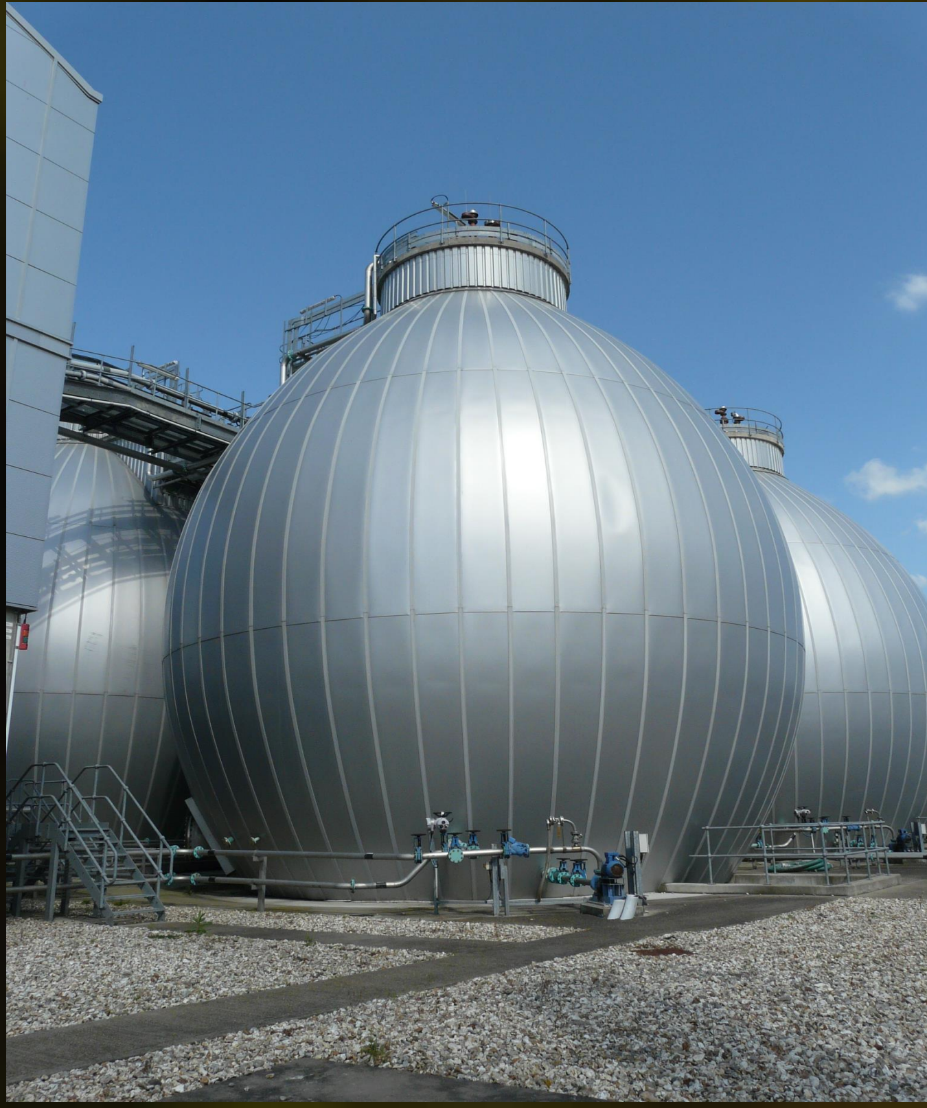
Sewage sludge anaerobic digesters
