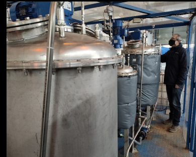
Figure 3: Pilot plant for bio-H 2 production.
