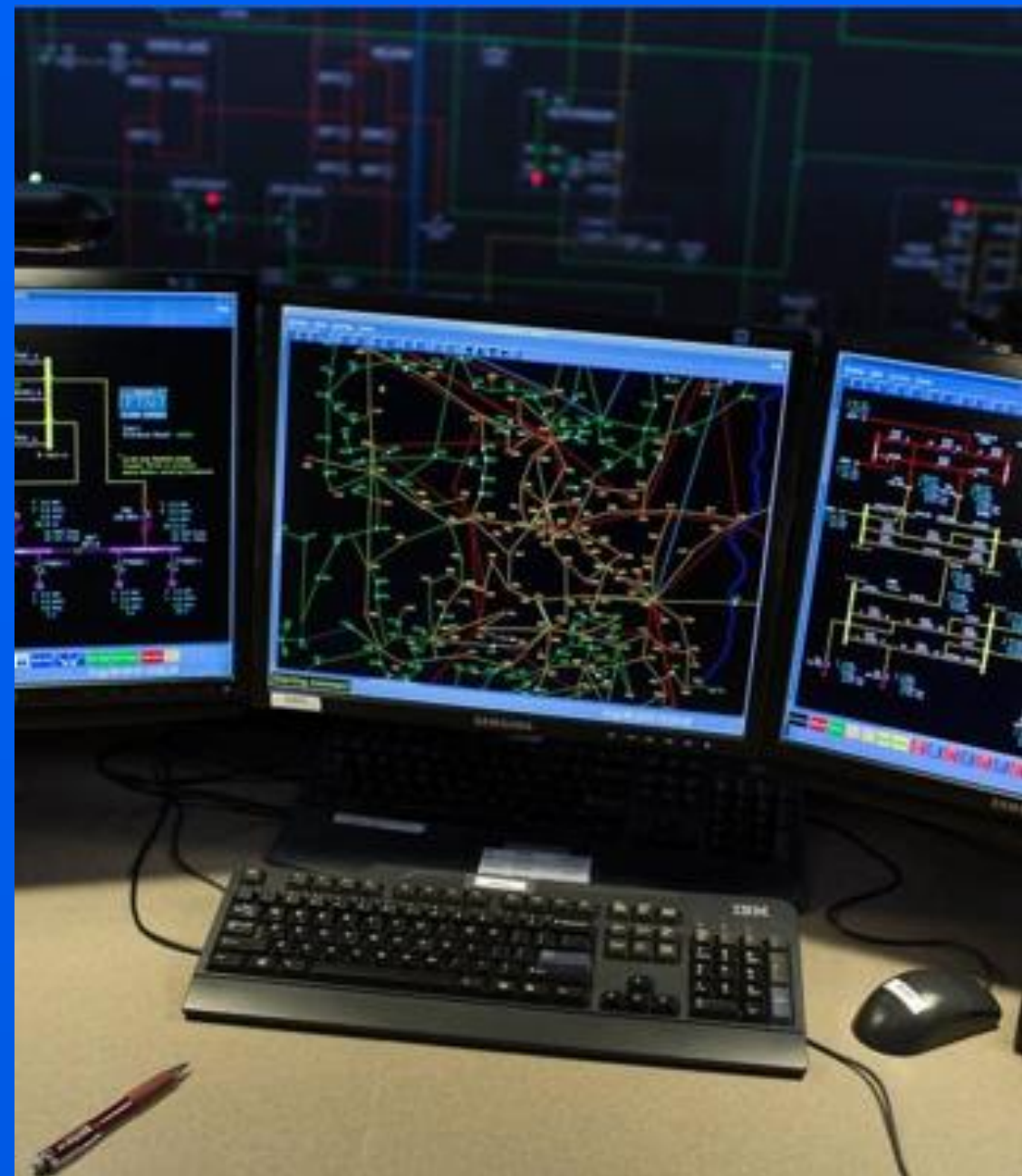
Figure 1: Energy control centre
