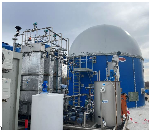
Figure 2. a) FWDs implemented in the demo plant and b) food waste dosing and AnMBR systems in the Valdebebas WRRF
