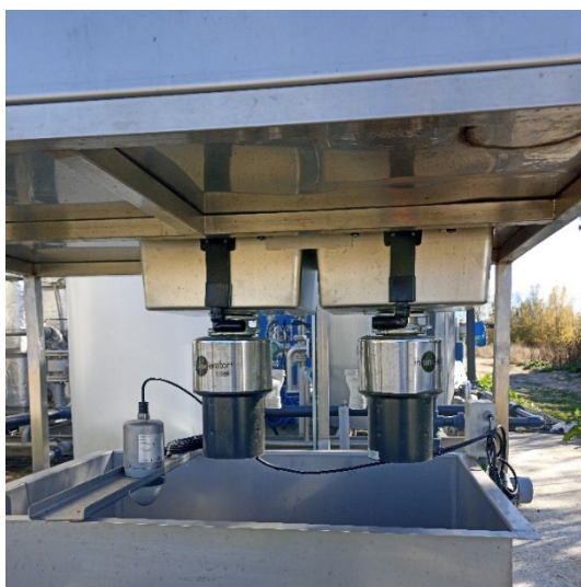
Figure 2. a) FWDs implemented in the demo plant and b) food waste dosing and AnMBR systems in the Valdebebas WRRF
