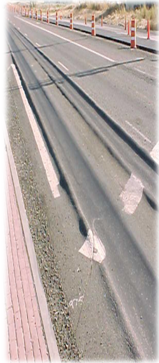
Modified asphalt mixture with crumb rubber and 50% RAP
