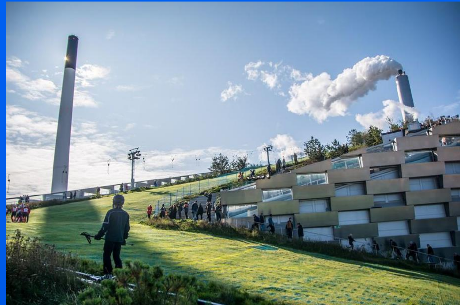
Figure 1: Waste-to-Energy plant in Copenhagen
