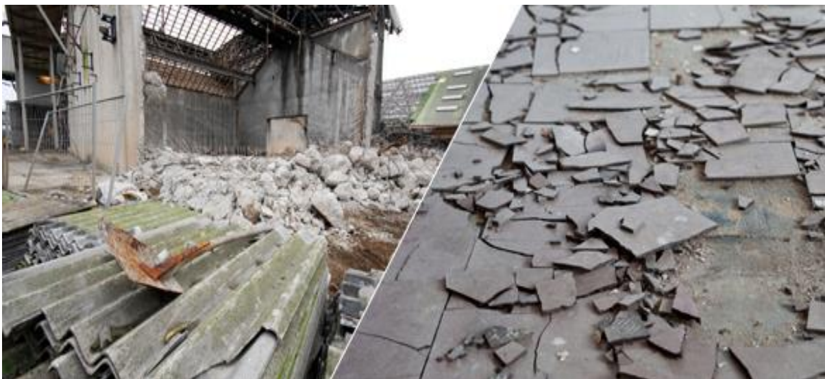
Figure 1. Asbestos in debris [2]
