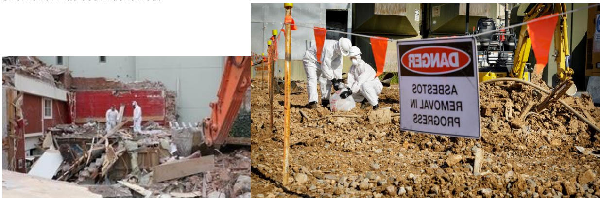
Figure 4 Work on rehabilitation when asbestos is identified [10]
