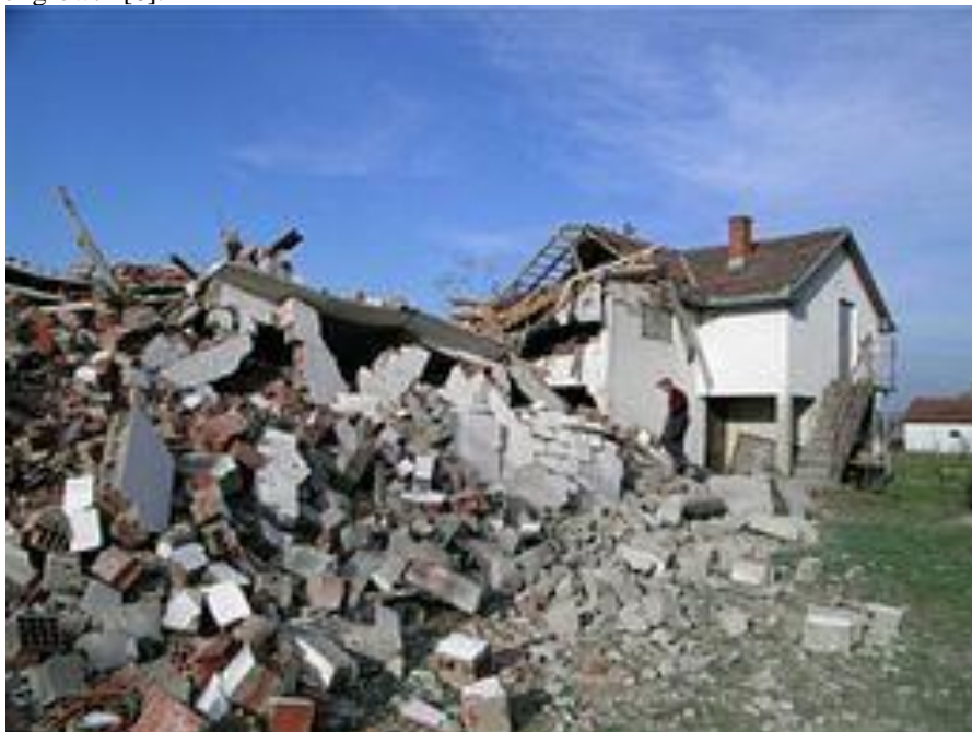
Figure 3 Kraljevo after the 2010 earthquake [5]
