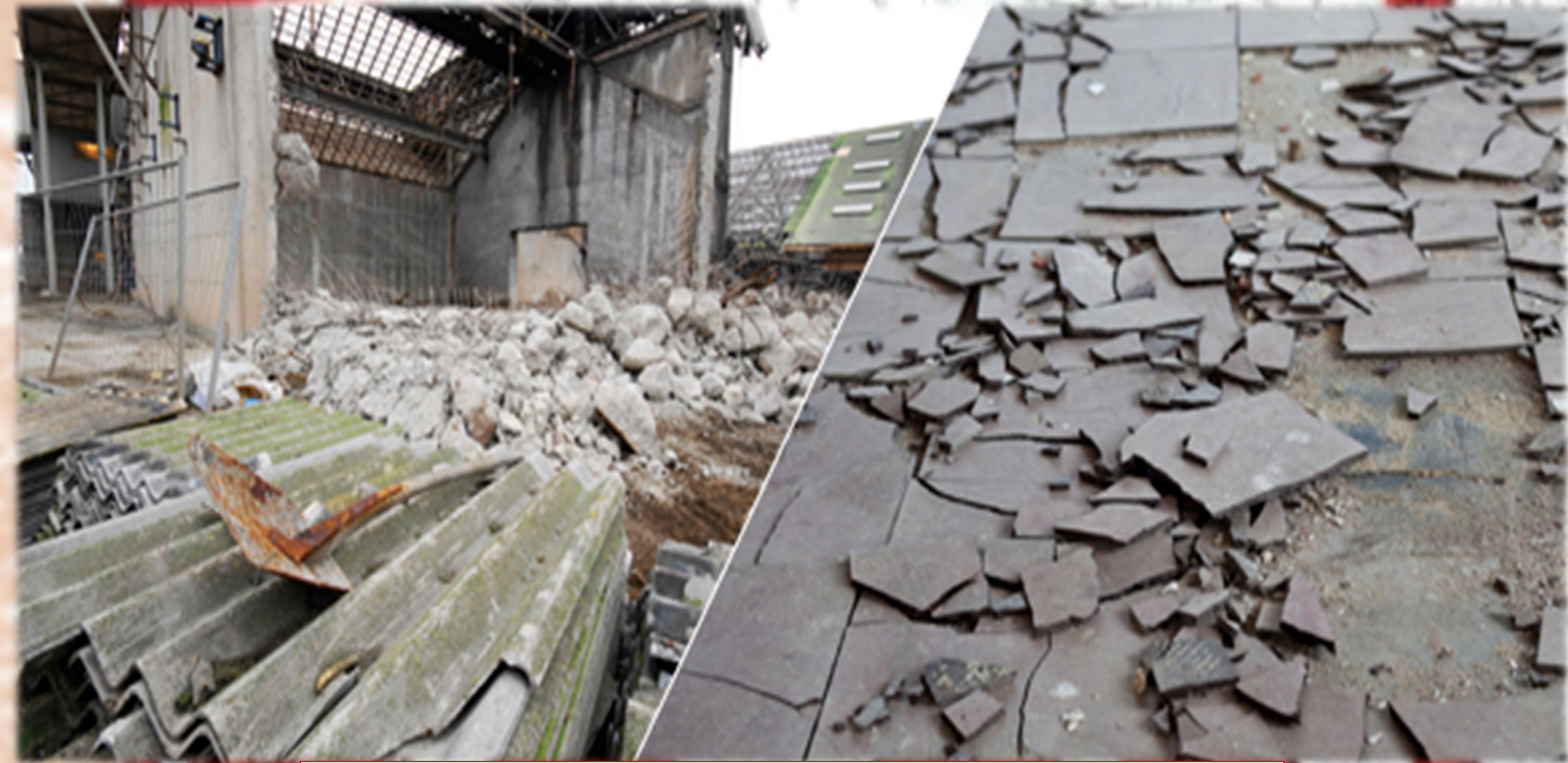
Fig. 1 Asbestos materials after disaster
