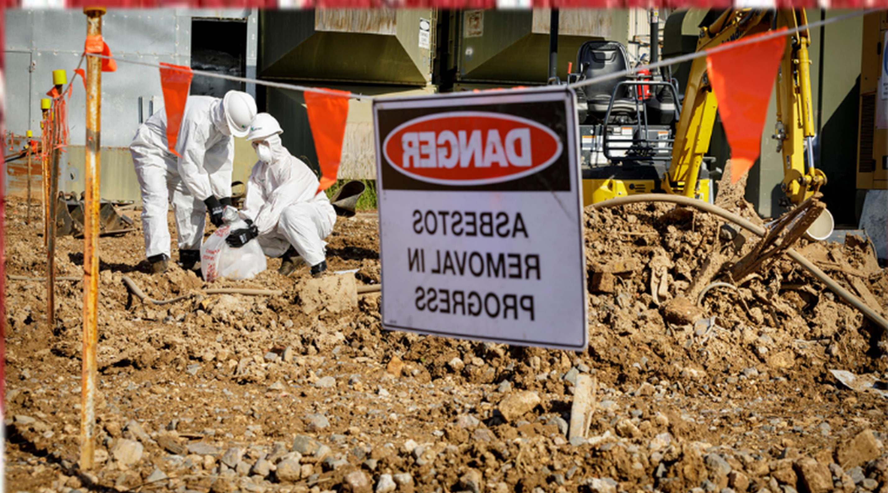
Fig. 3 Work with asbestos waste
