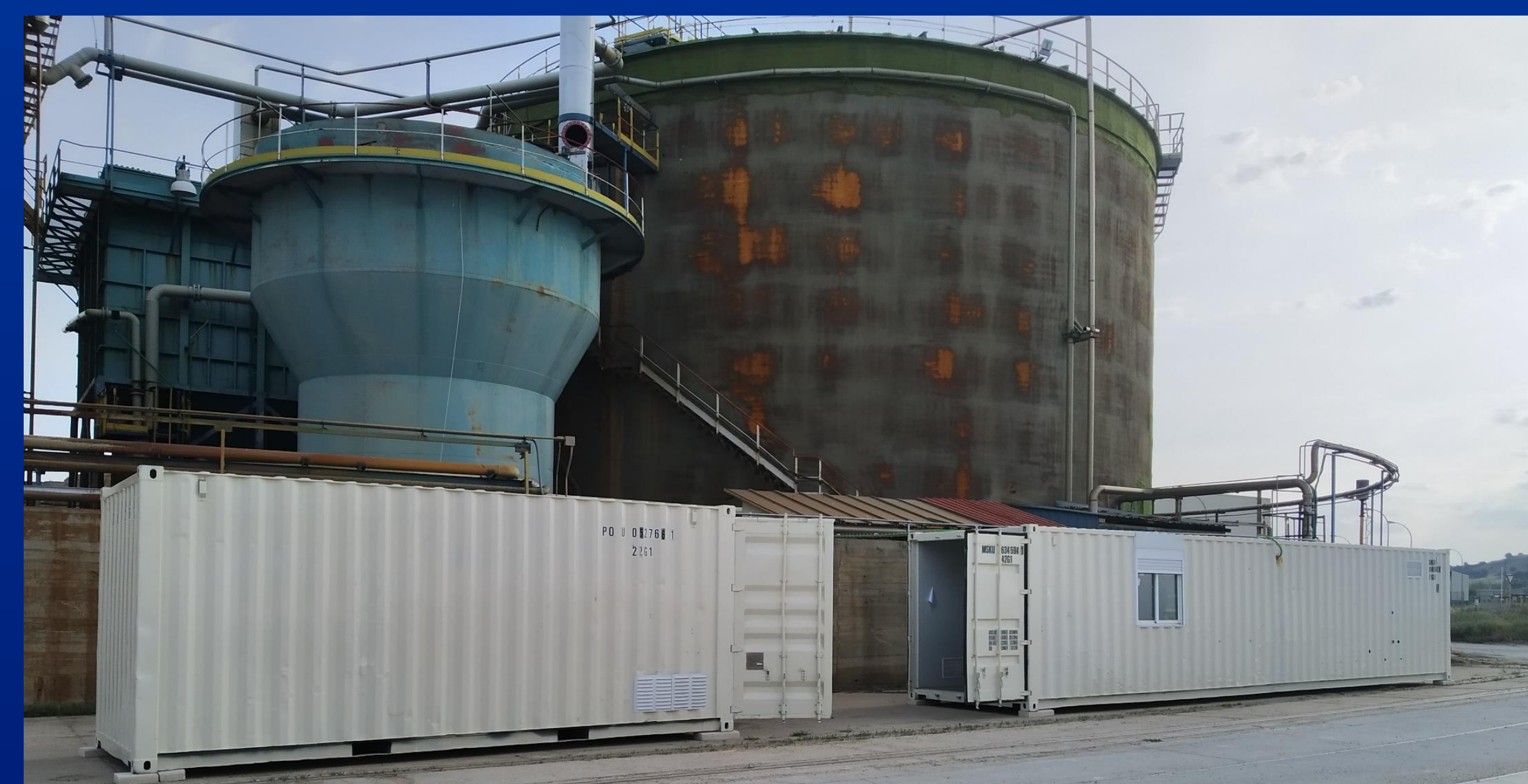
Figure 5: Biogas upgrading pilot plant
