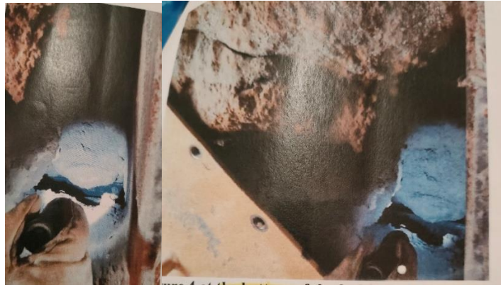
Figure 18 C 2 nd and 3 rd part boiler ash formation causing blockages
