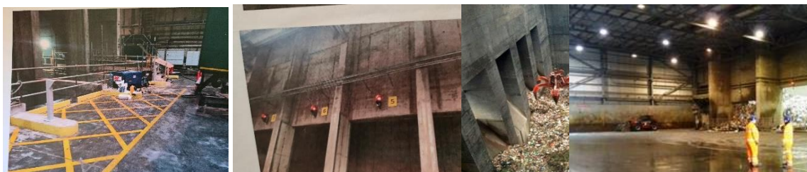
Figure 8A A view inside the Tipping hall area encompassing a Traffic Management System linked to appropriate unloading bays with raised kerbs. The unloading of waste is assisted by the traffic controller system thereby instructing drivers when and where to unload waste. Vehicles are directed to the appropriate bay using traffic light indicators.
