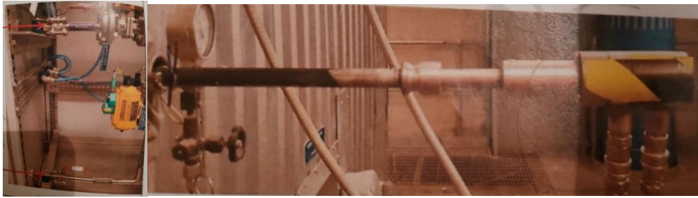
Figure 11B SNCR dosing system, lances and associated features
